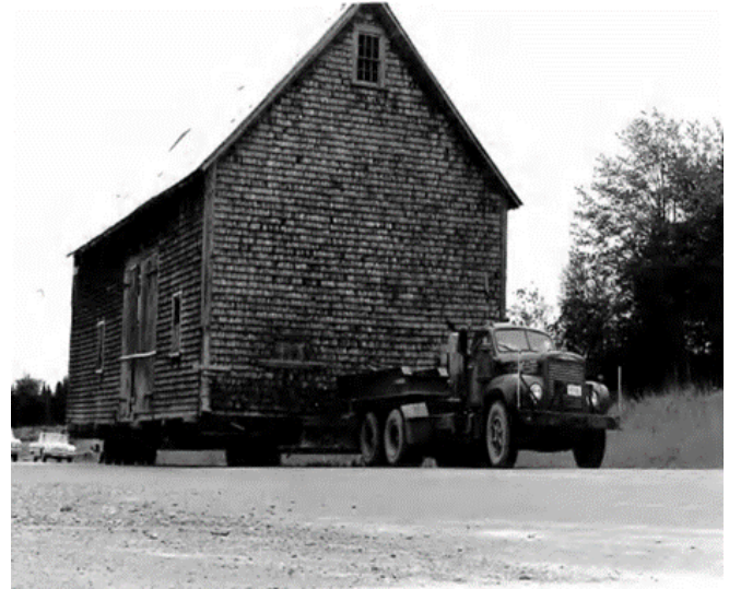
Joslin Barn being moved 1969
