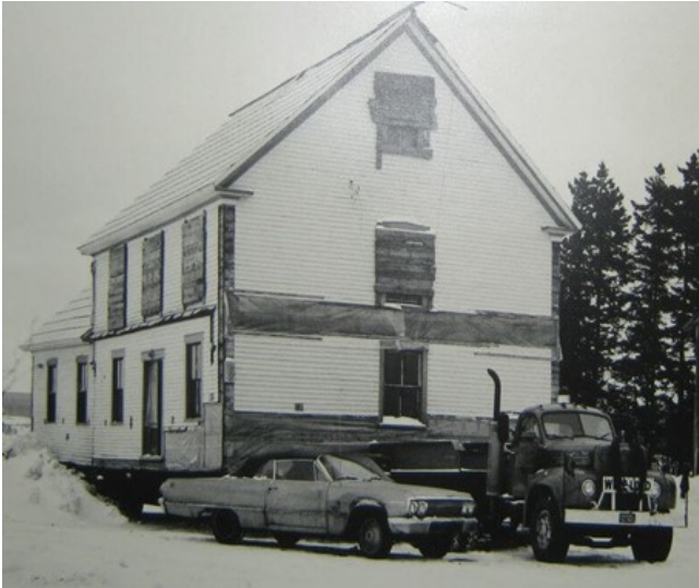
Joslin House being moved 1969
